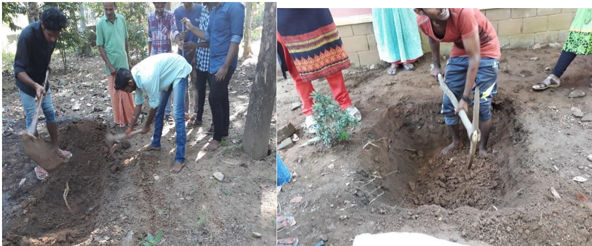
WATER RECHARGING PIT MAKING @VILLAGE
